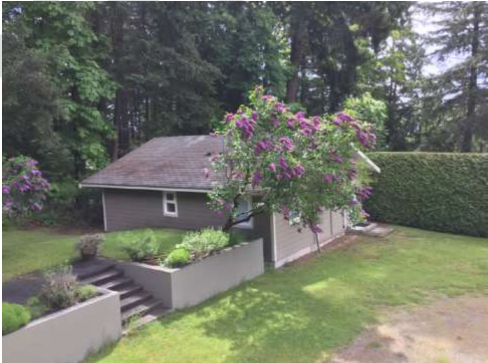
View of Accessory Building from Principal Dwelling
