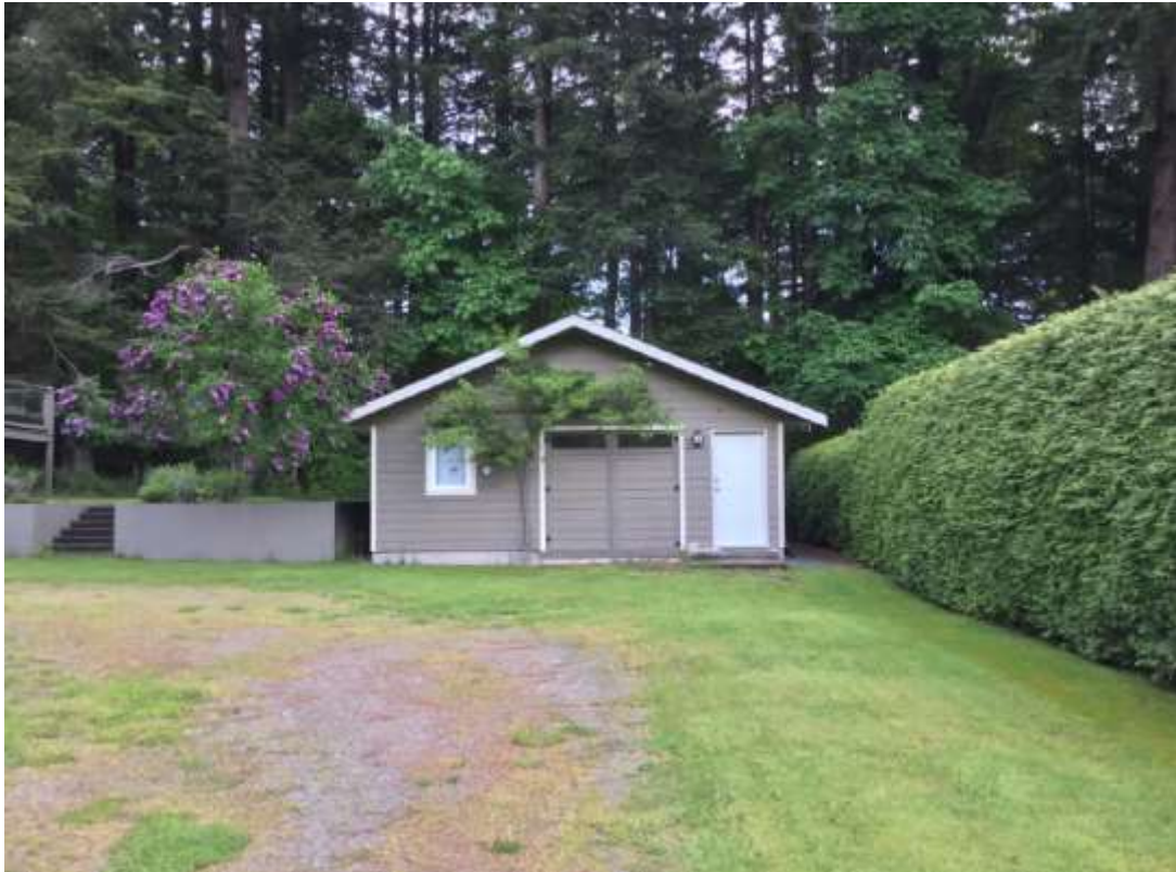
Figure 4: View of Accessory Building from Croteau Road
